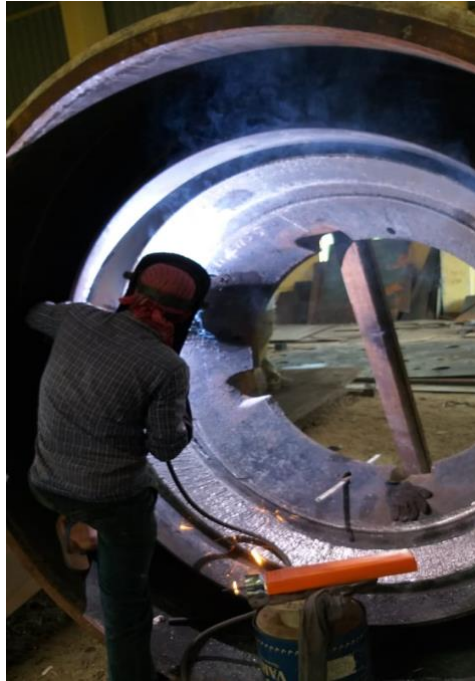
PHOTO- C (Welding in progress)
