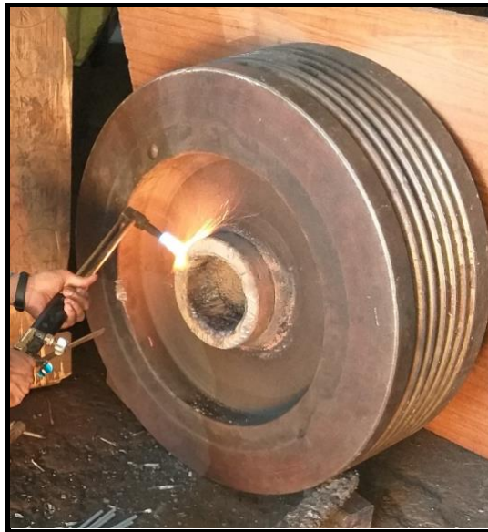
PHOTO- D (Preheating in progress)
