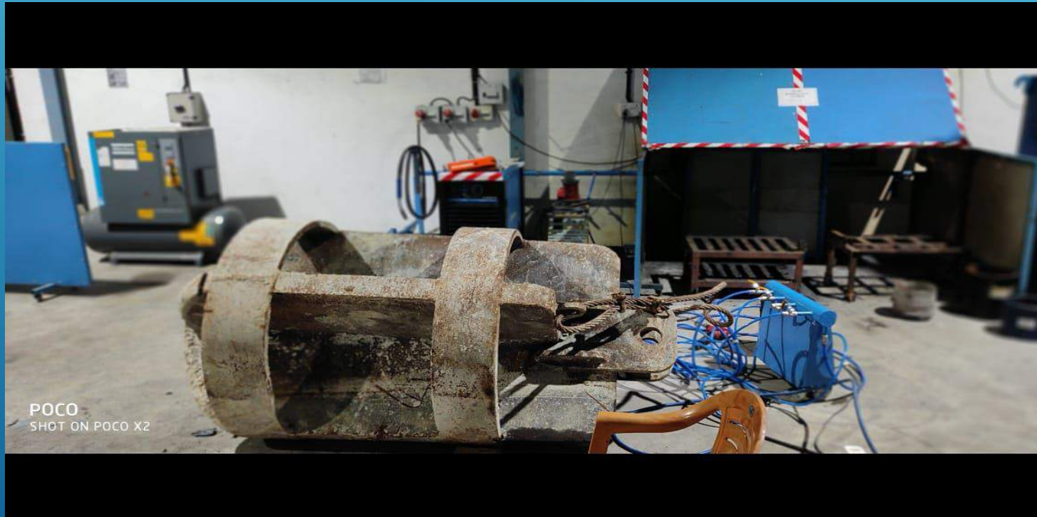
REPAIR IN PROGRESS Photo: 5
