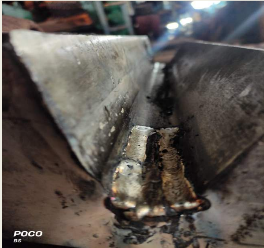
Photo:05 - Removed the crack by Gouging Method
