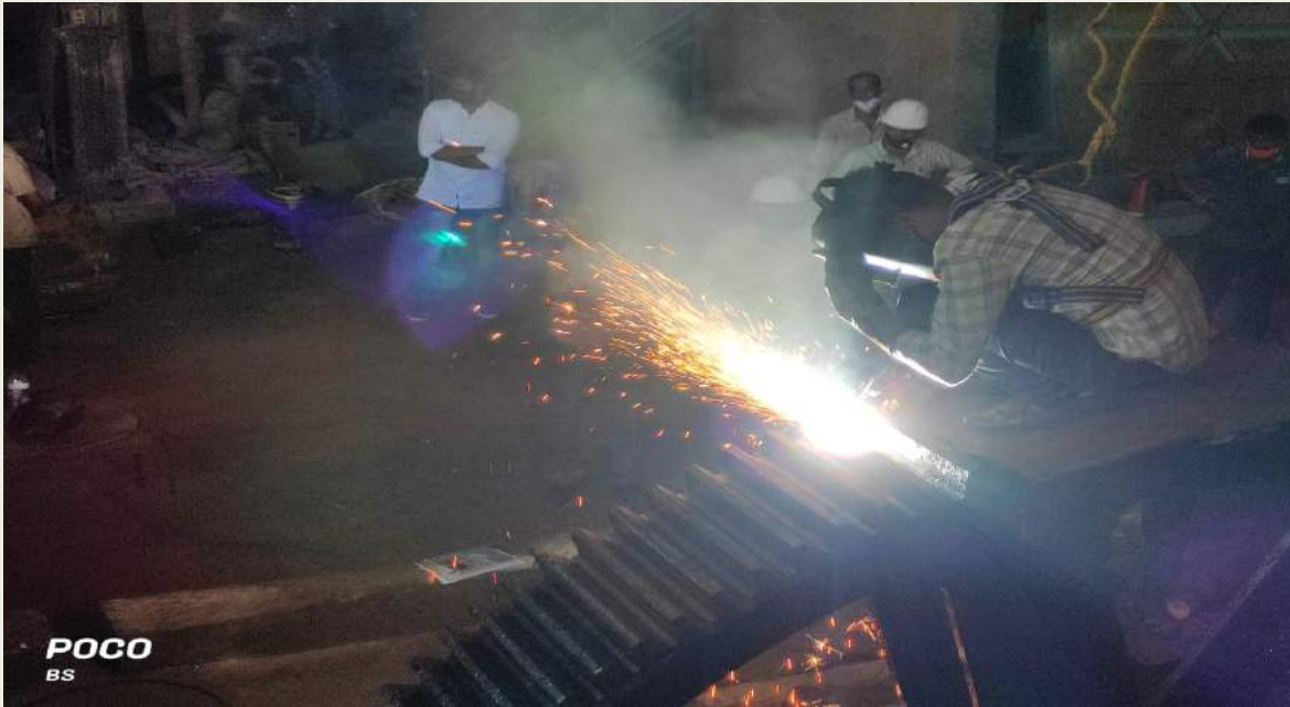
Photo: 06 -Doing a Welding on Gouged area
