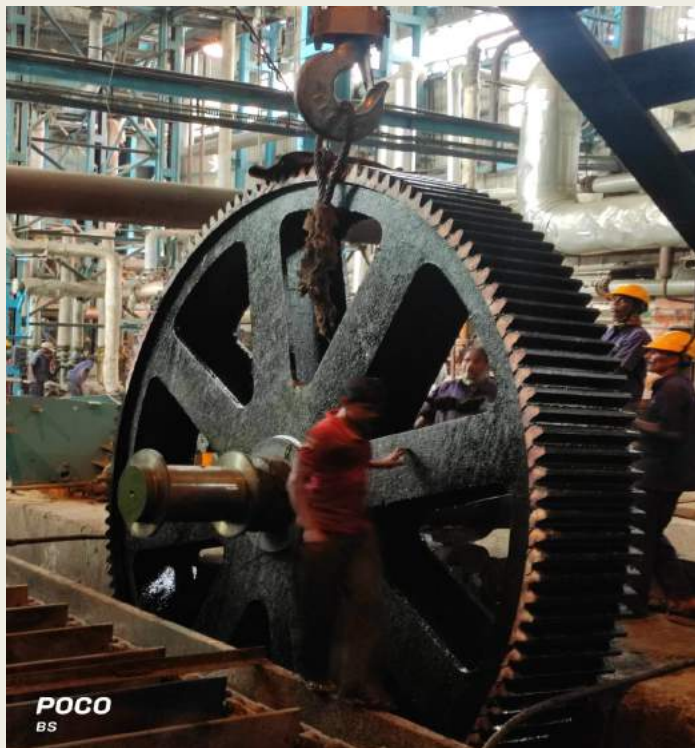
Photo:02 - Lifting the Gear
