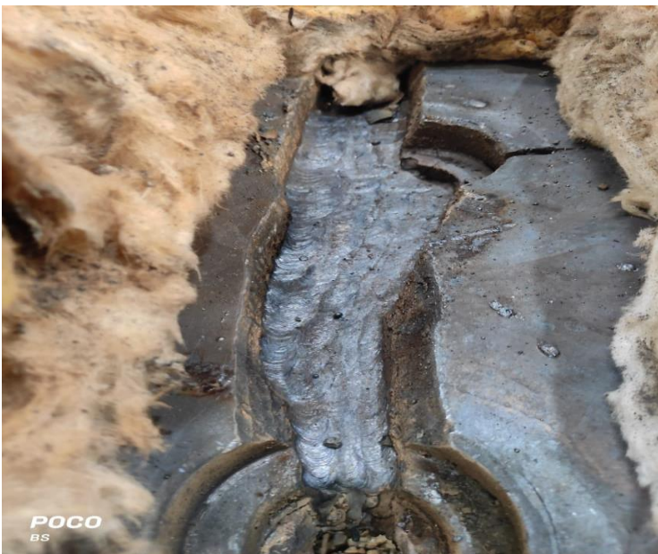
Photo: 06 - Welding on Gouged area
